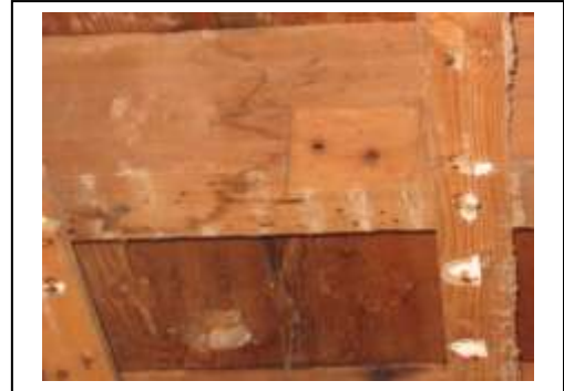
Joinery Evidence of Partition Wall.
