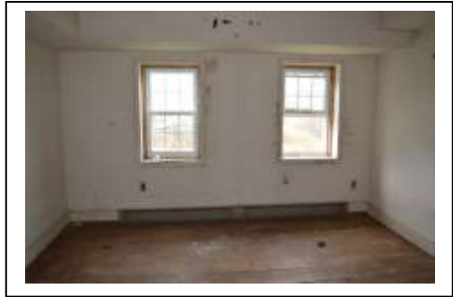
West Corner Room Showing Boxed Ceiling.
