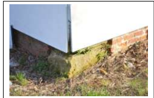
South Corner Sandstone Blocks and Brick Infill.
