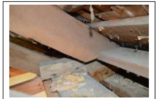
Roof Rafters and False Plate.
