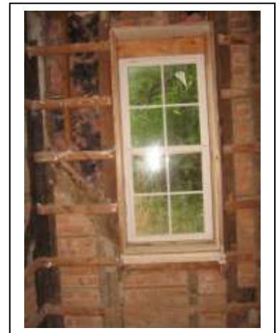
West Corner Gable Window.
