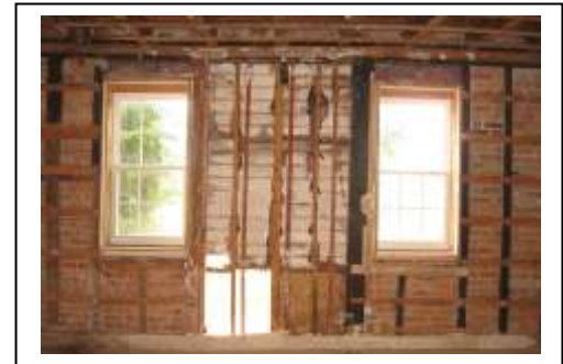
Front Wall Framing.
