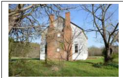
Northwest Gable End Chimney.
