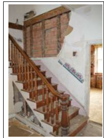
Stairs and Brick Nogging.
