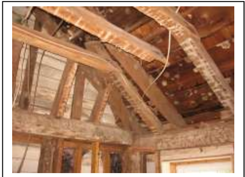
Vaulted Ceiling Frame Members.
