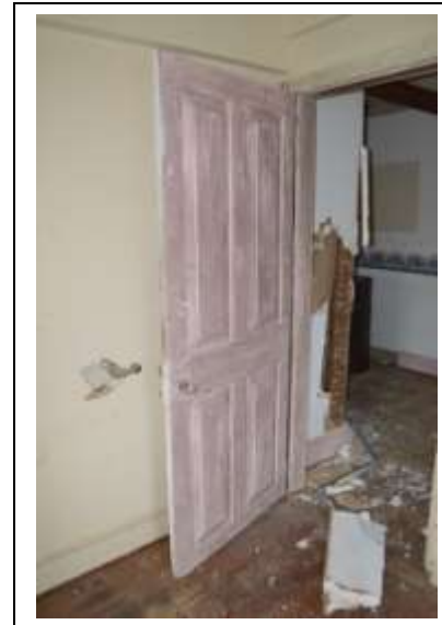
Typical Second Floor Door.
