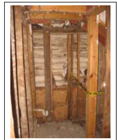
Mortise Joints on Front Sill Plate.
