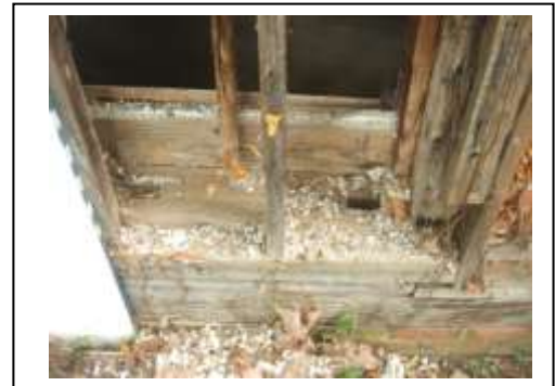
Mortise Joints on Front Sill Plate.
