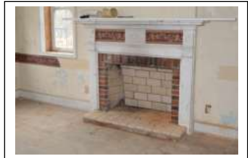
Main Room Fireplace.
