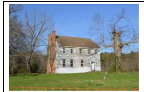
Southwest Façade (Front Façade).
