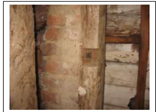
Evidence of Chimney and Mantle on Southeast Gable Wall.
