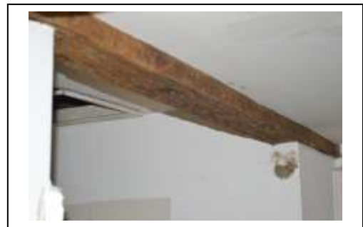
Exposed Beam in Second Story Hall.
